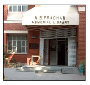
Two iron grating covers have been placed as foot mats. These can trap front wheels of a wheelchair as well as white cane and the collapsible gate's threshold poses a trip hazard for everybody.
